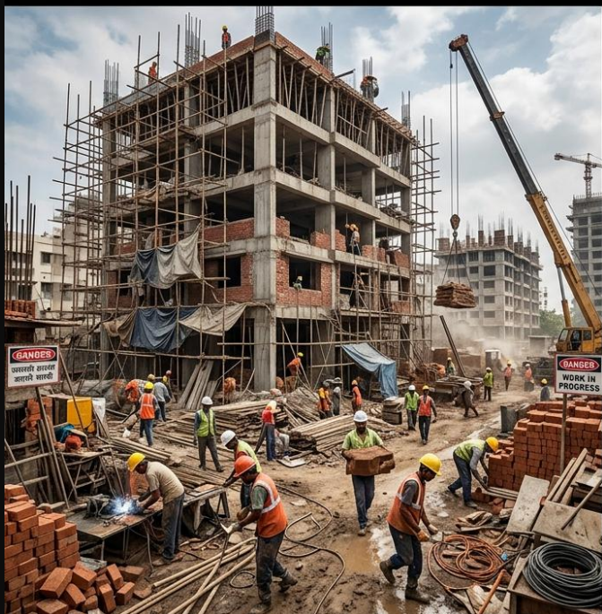
CHAOTIC TRADITIONAL CONSTRUCTION SITE
